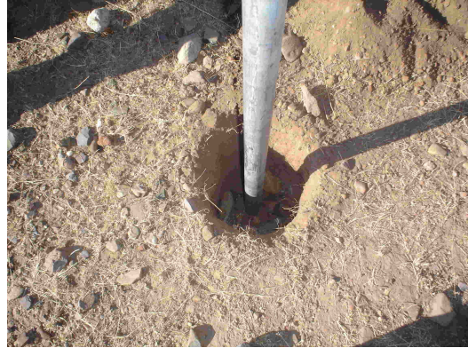
Figure 23: a) Soil digger recommend for post installation .b) Installation of metal pipes in the field .c) Final result.
