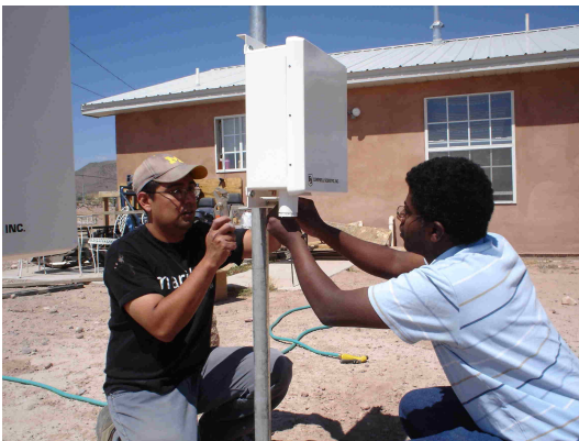
Figure 24: a) Fixation of the enclosure to the post. b) Final result
