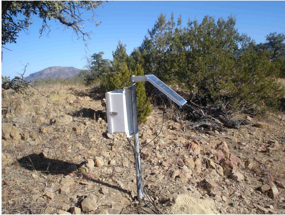
Figure 25: Solar panel Installation
