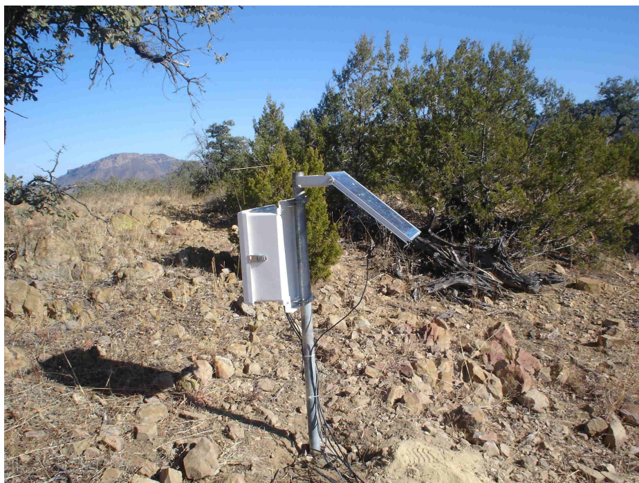
Figure 55: Solar panel Installation
