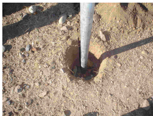
Figure 53: a) Soil digger recommend for post installation .b) Installation of metal pipes in the field .c) Final result.
