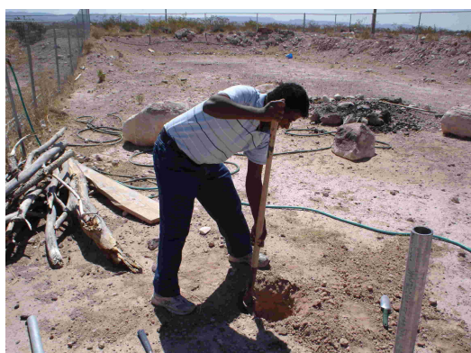
Figure 53: a) Soil digger recommend for post installation .b) Installation of metal pipes in the field .c) Final result.
